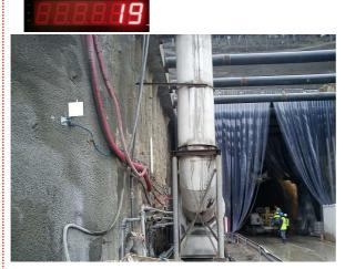
A long-range RFID tag fixed to people's helmets can be used to detect the direction of their movement as they pass in front of the reader terminal, without any action on their part.
